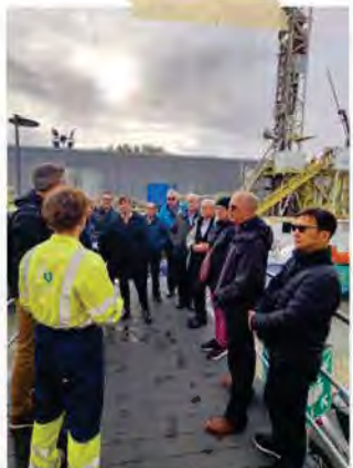
Geothermal Well site visit by ES BOD and team, Delft University of Technology
